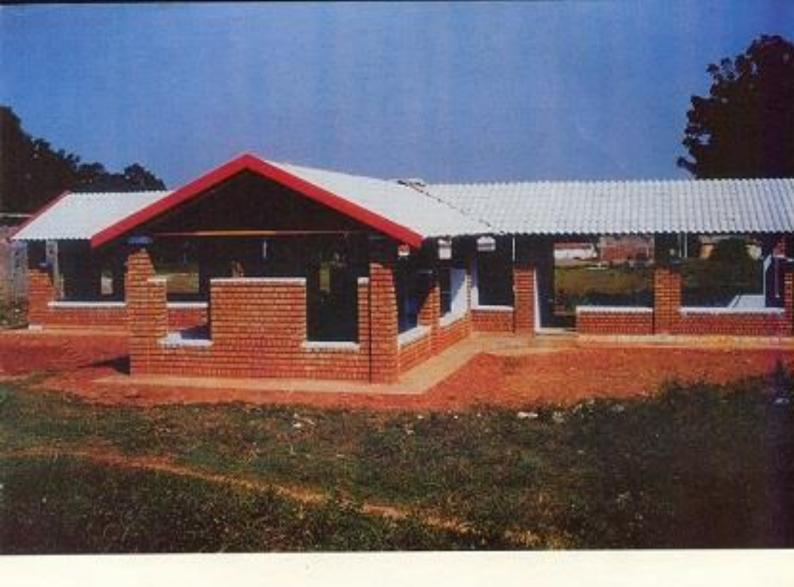
uniformity. Without in any way compromising on standards of safety, the majority of the designs cut down on cement, steel and shuttering by making a more efficient use of these materials. This meant a remarkable overall saving on each building of almost 30%.
