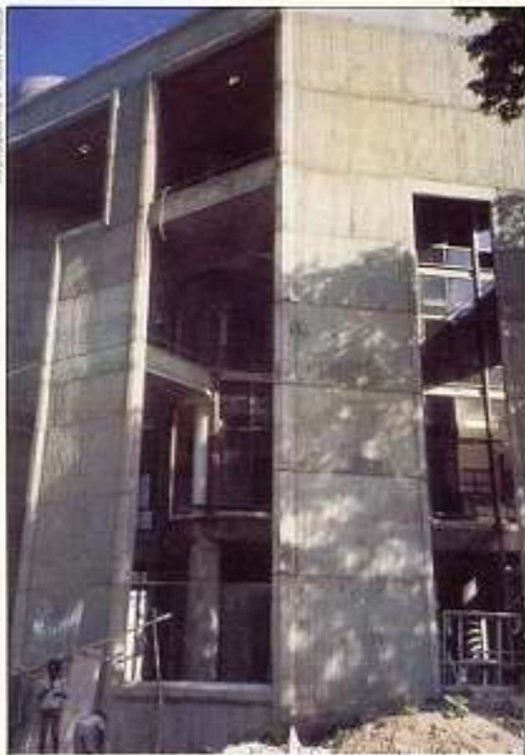
Above Openings in the screen give views of the glass-wrapped office work.
