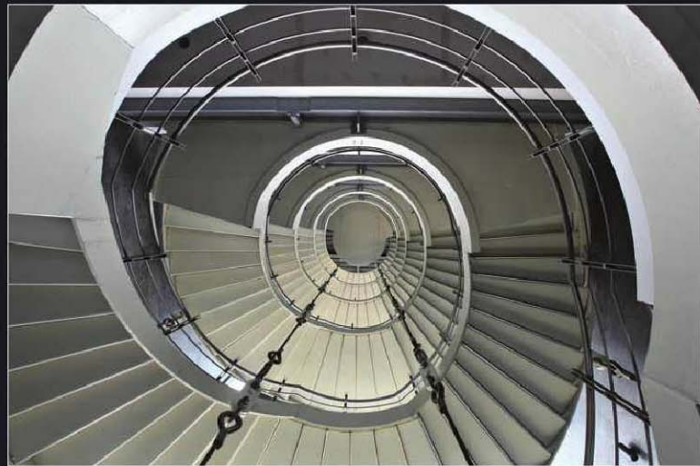
the 30 mm cables suspend the 'staircase' from the roof
