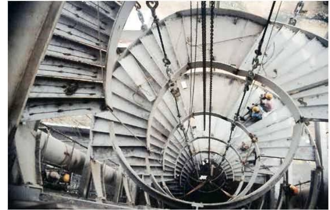
The spiral staircase during the construction stage
