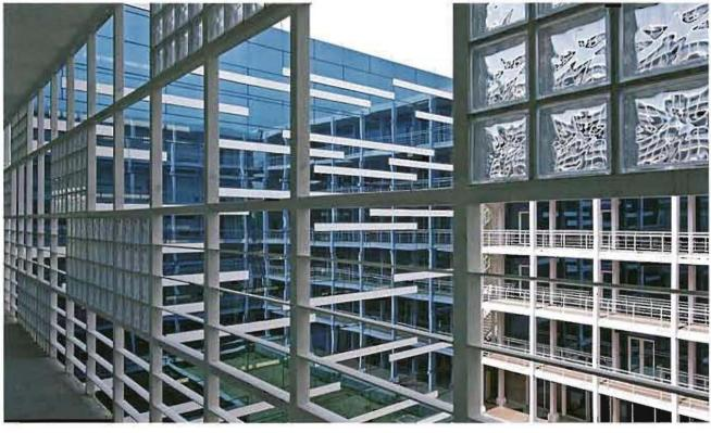
The surface itself forms the structure of the building as structural glass, reinforced concrete frames, structural steel staircases and corridors emerge and disappear, separate and connect to map the programmatic and contextual elements
